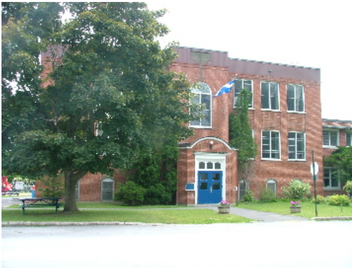
Butler Elementary School
